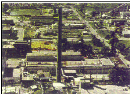
Building 3019A, Radiochemical Development Facility, currently stores the U-233 to be processed under the Request For Proposal
